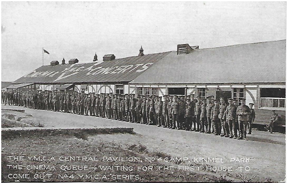
Fig 6 A post card view of the Central Pavilion in Number 4 Camp
