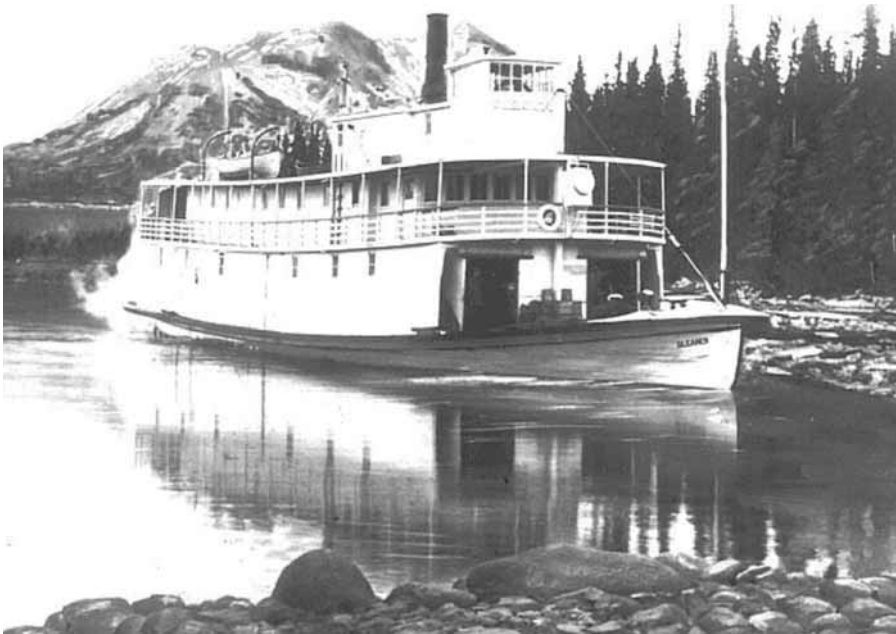
Fig 8 Gleana built in 1899 at Lake Bennett which received the mail contract the same year.
