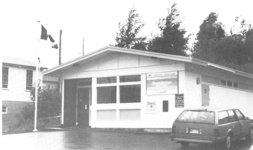
Fig. 4 Post Office at Shoals Harbour
